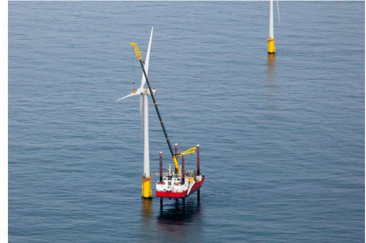
Maintenance of offshore wind turbine
